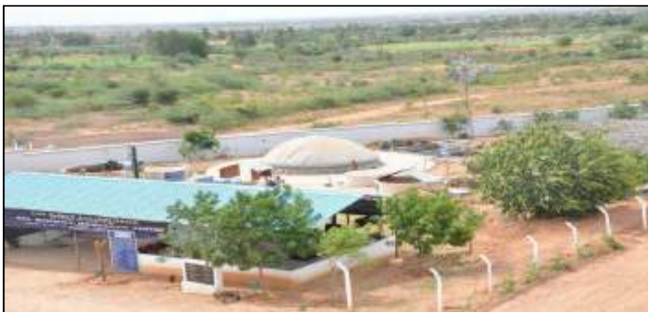
An aerial view of the Biomethanisation plant. The gas production capacity of the plant is 500m 3 /day. Utilizing this gas the power produced is 60 kwe / hr. The digested material is converted into nutrient rich soil conditioner through vermicomposting process.
